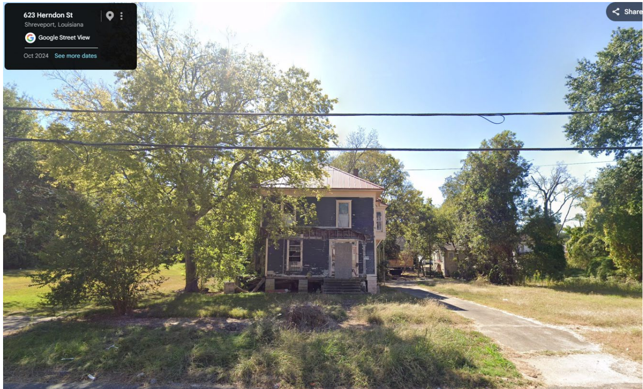
Exhibit A. Front Facade View
