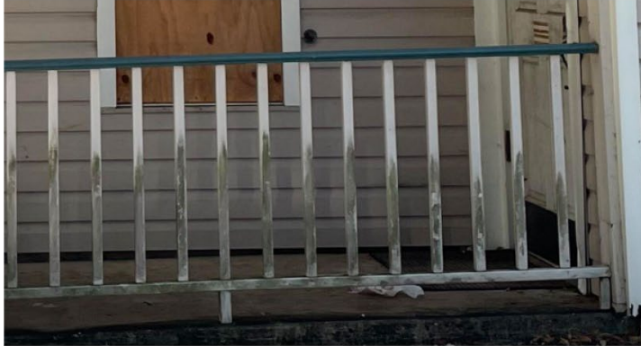
Fig: Existing Handrails at the porch
