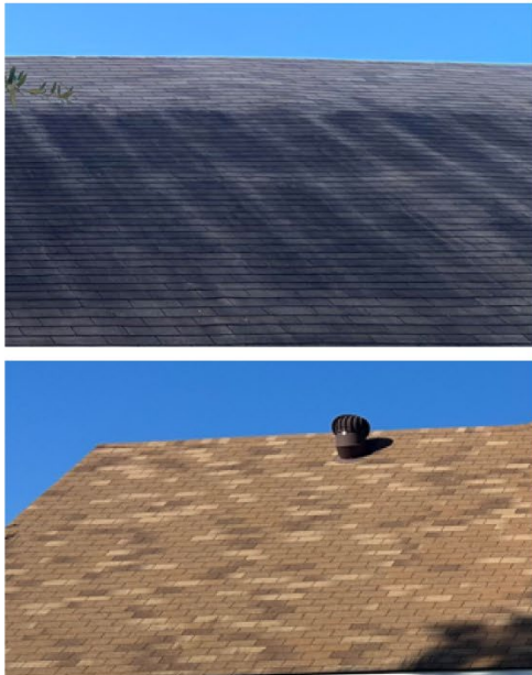
Fig: Existing Roof
