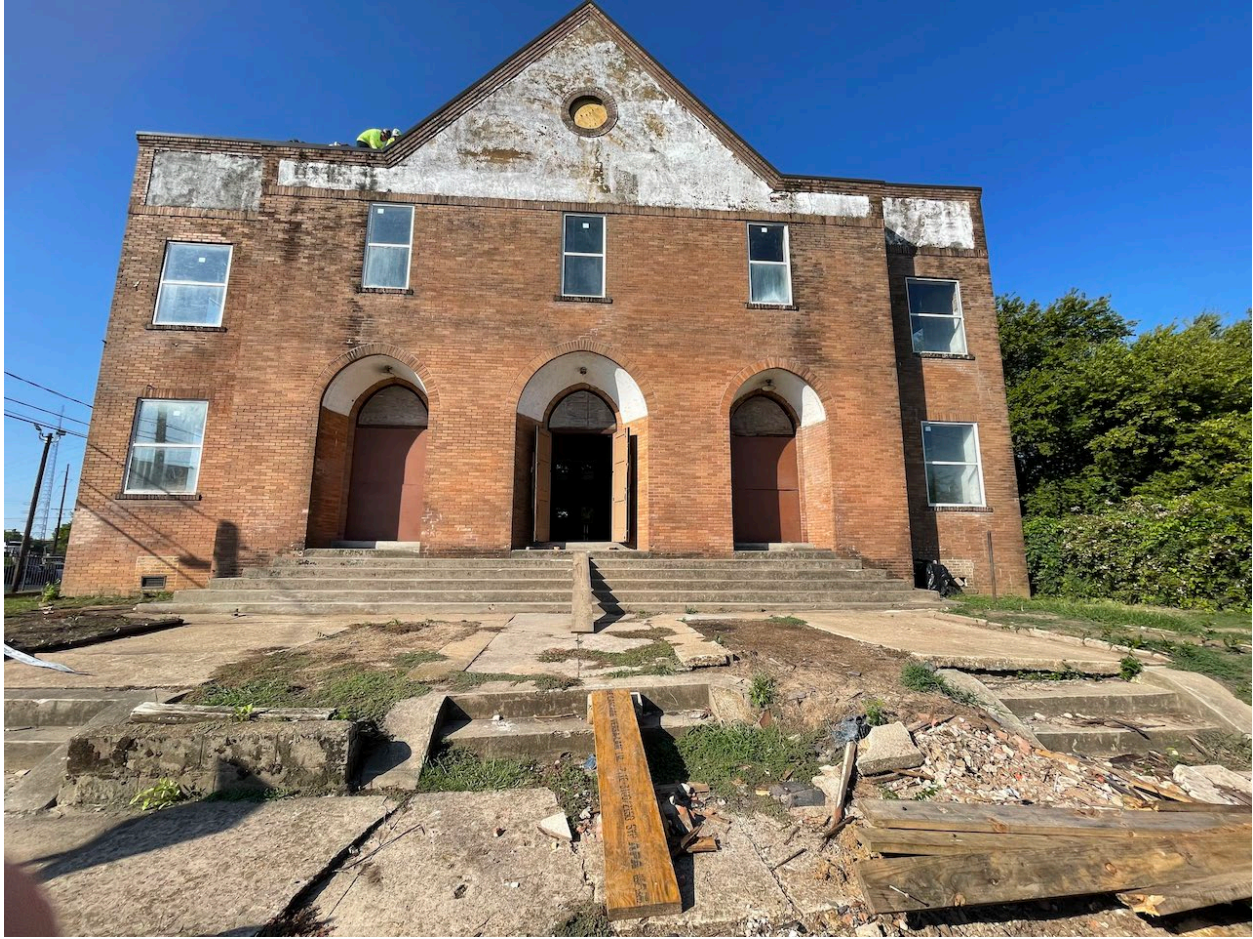
Figure 1 - Front Concrete Walkway Repair
