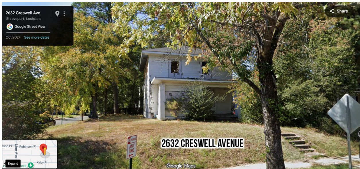
Exhibit A. Front Facade View
