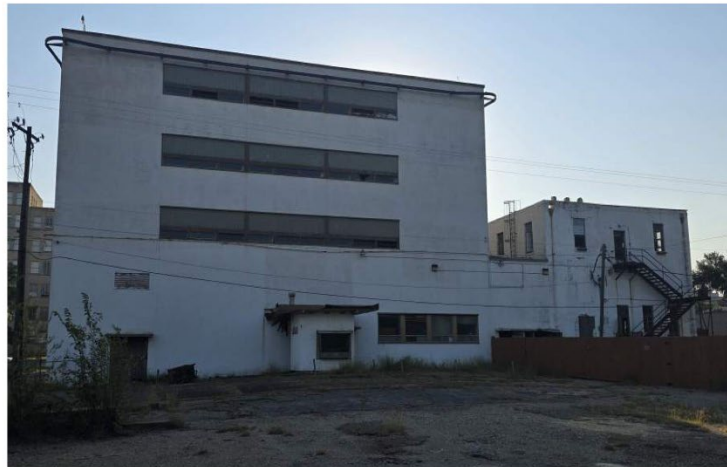
Exhibit G - Existing Conditions Photograph - Rear Elevation
