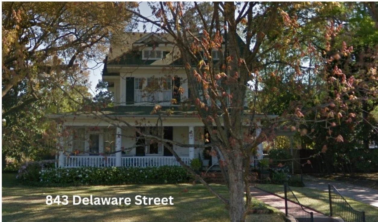
Exhibit A. Front Facade View
