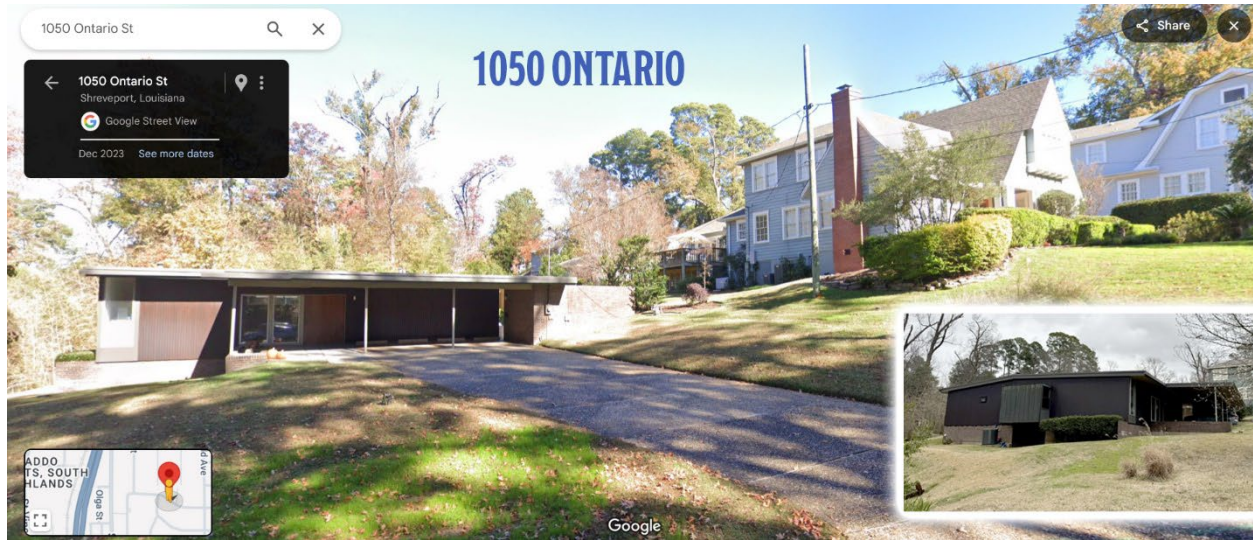
Figure 1 - 1050 Ontario Street, American Modernist residence - Simon Herold House in Shreveport
