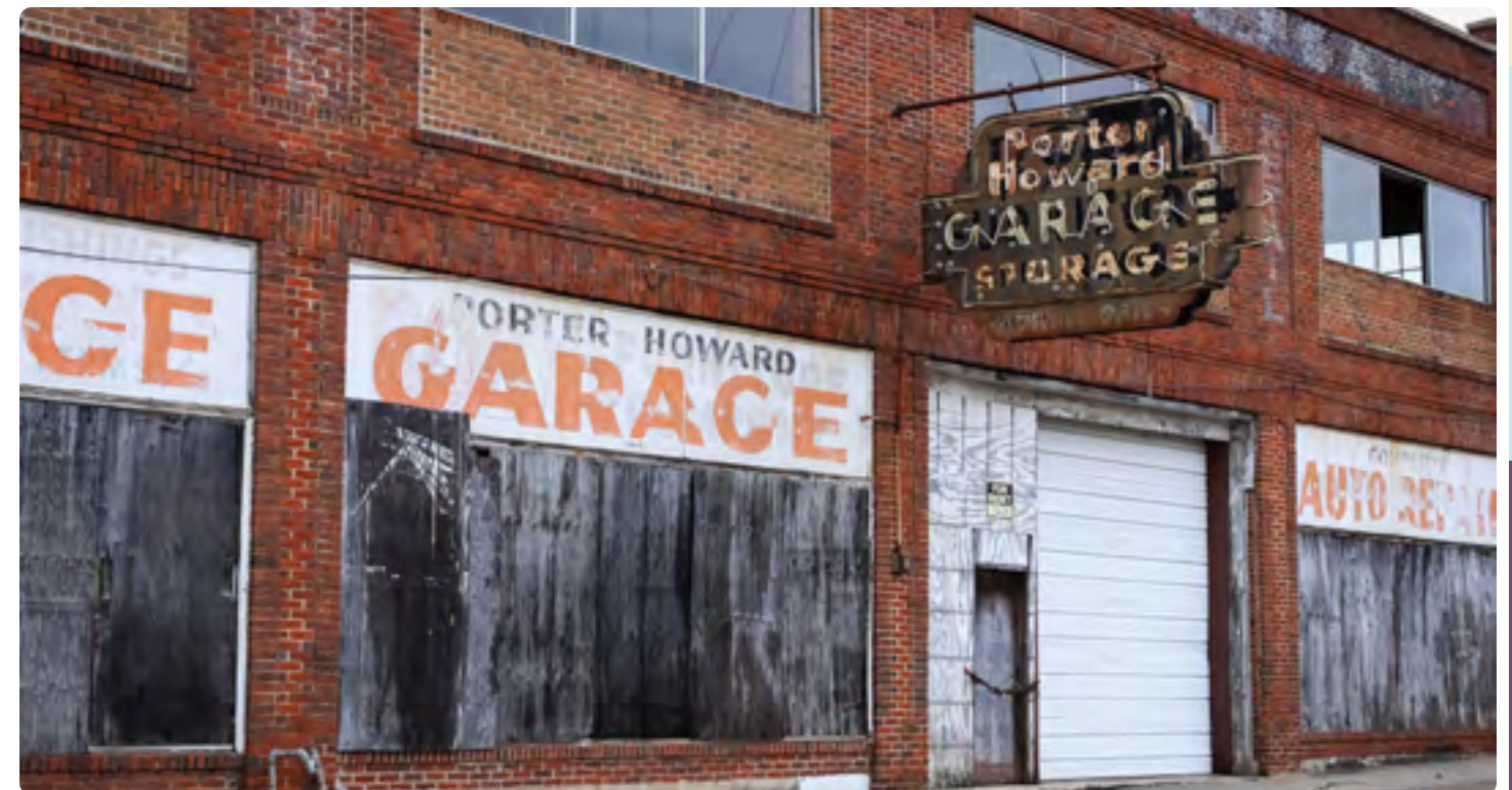
SIRA can facilitate the reuse of vacant and abandoned properties, including residential, commercial, and industrial buildings and land. Source: Sabrina Gordon | Dreamstime.com
