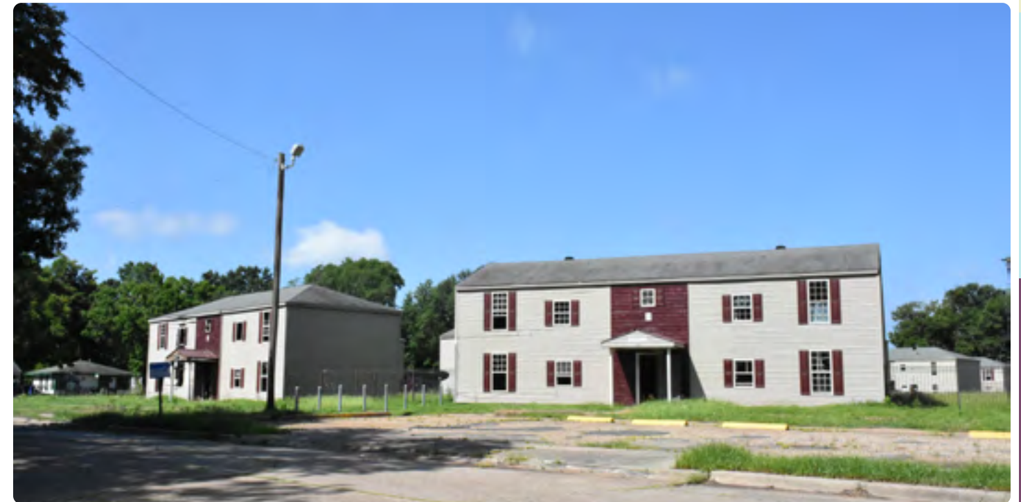
The Silver Lake/Woodlawn Apartments in the Cedar Grove area are a visible example of neglect and blight. Source: Asakura Robinson
