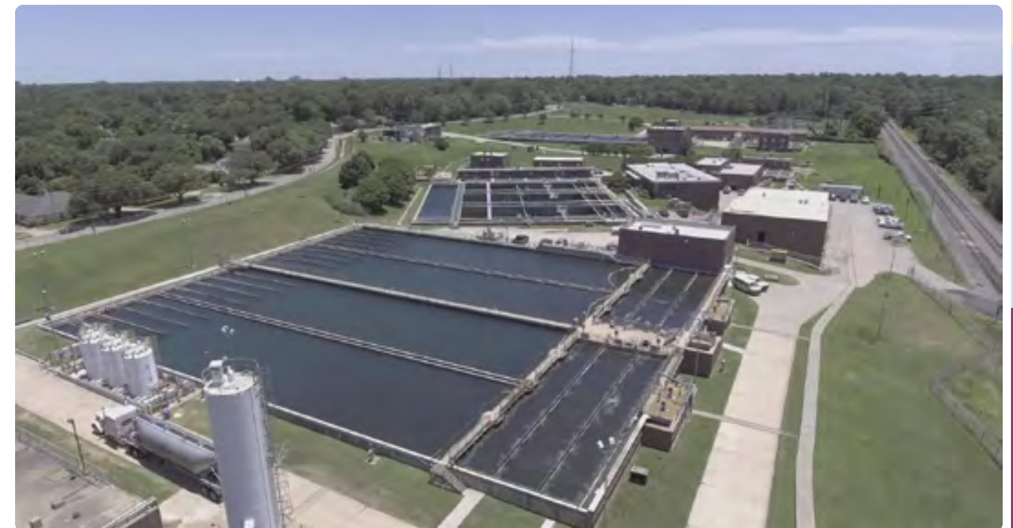
T.L. Amiss Water Treatment Plant. Source: Clean Water Shreveport
