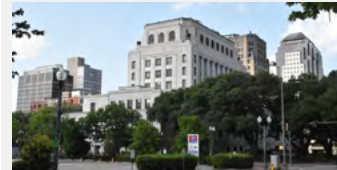
Caddo Parish Courthouse and skyline. Source: Asakura Robinson
