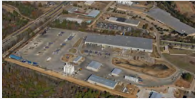
Valley View Drive. Source: Kevin Bryan Architect
